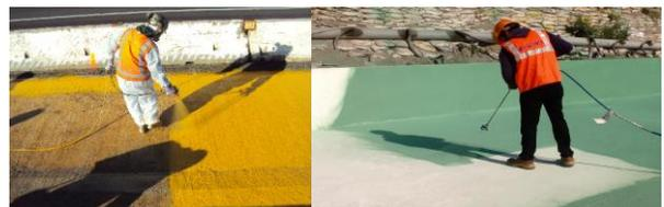
No 'pre-striping' of existing cracks required, Monolithic, Excellent wear resistance, UV & weather resistant , Attractive appearance , Very low dirt retention , Easy to
